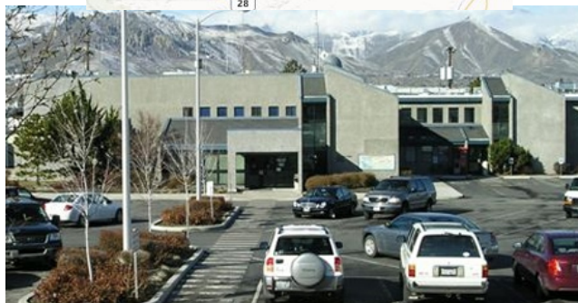
One site of the Douglas County District Court.
