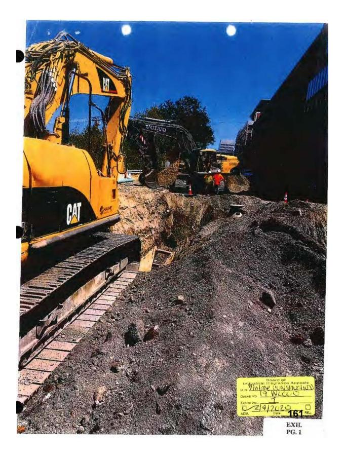
The Board also observed that "[t]he photograph shows excavation debris placed immediately next to the excavation, thus making the total depth to the top of the trench shoring box even higher than the surrounding street surface." CP at 3-4.
