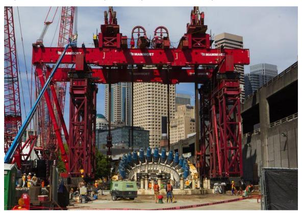
After a 2013 breakdown, the tunnel-boring machine Bertha was taken apart and put back together. Here, workers in 2015 watch the 57.5-foot diameter cutter head and drive unit being rotated into a vertical position to then be lowered into a pit for reassembly. Bertha didn't resume digging until 2016 and broke through next to Seattle Center in April 2017. (Ellen M. Banner / The Seattle Times, file)
